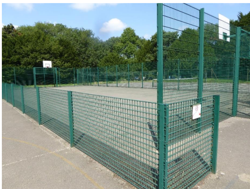
Tattenham Recreation Ground MUGA
