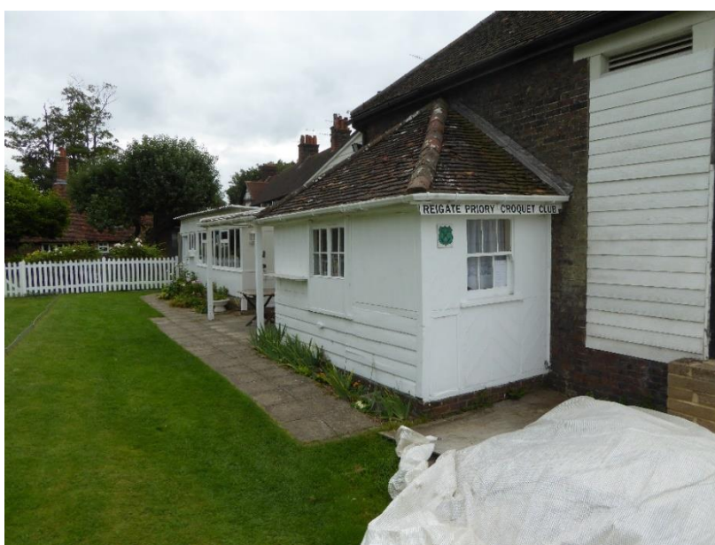
Reigate Priory Croquet Club pavilion
